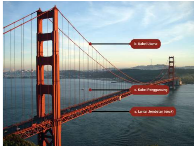
Gambar 3.13 Jembatan gantung ( suspension bridge ) Sumber: www.smhlawmed.net /Rizal Abdi (2021)
